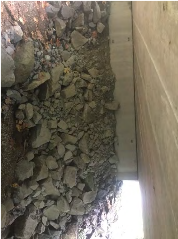
Left Bank Abutment when facing downstream
